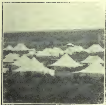
On railway construction, Western Canada, 1908.
